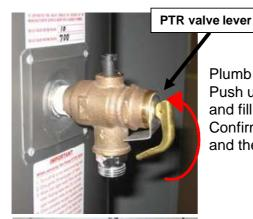
Plumb pipes to Storage Tank Unit and Heat Pump Unit. Push up the lever on the PTR valve to open, and fill in the tank with water.
